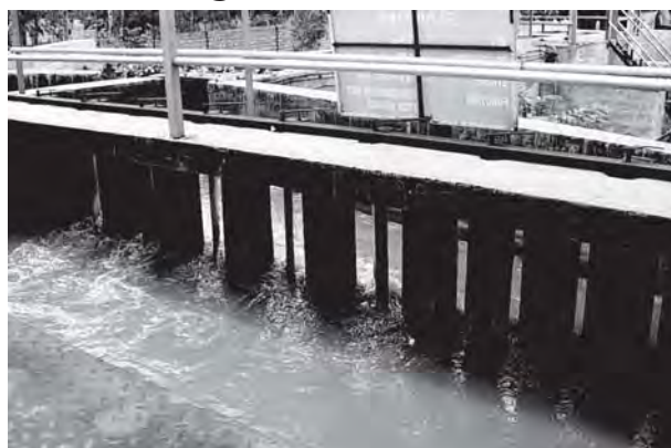
Fig. 18.4 Grit and sand removal tank
