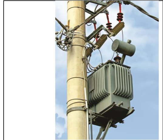
Fig. 2.44: Input output terminals of transformer
