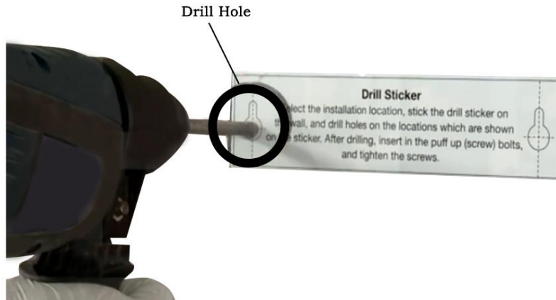
Fig. 3.90: Drilling on the wall
