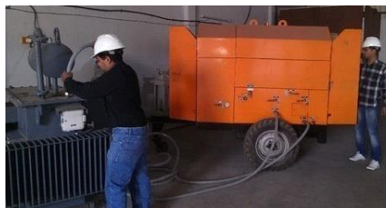
Fig.5.20 Filling of oil in the transformer using oil filling machine
