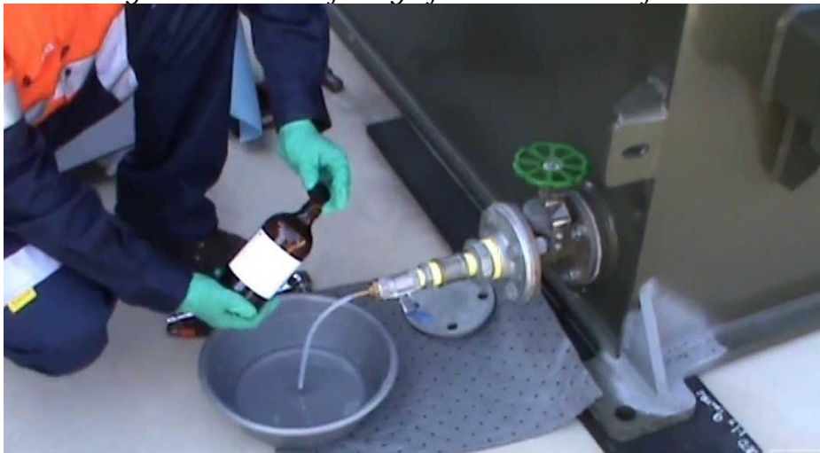
Fig.5.22 Replacing of oil from transformer
