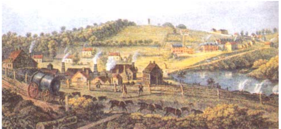
Caolbrookdale: blast-furnaces (left and centre) and charcoalovens (right); painting by F. Vivares, 1758
